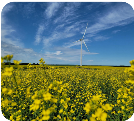
Bull Creek - 29.2 MW project located in the Municipal District of Provost, Alberta
