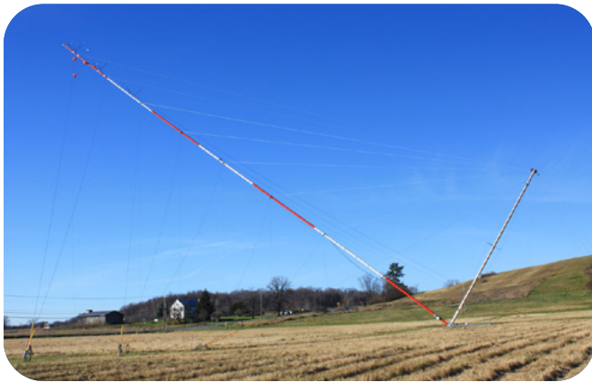
Photo of a met tower being installed
